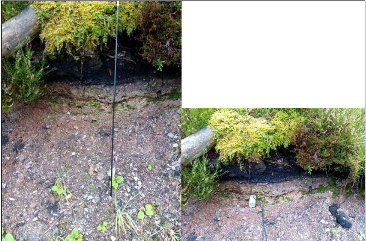
Figure 9.5: Turbine T49 & T50 soil profile exposing thin peat soil layer 0.1 – 0.4m thickness
