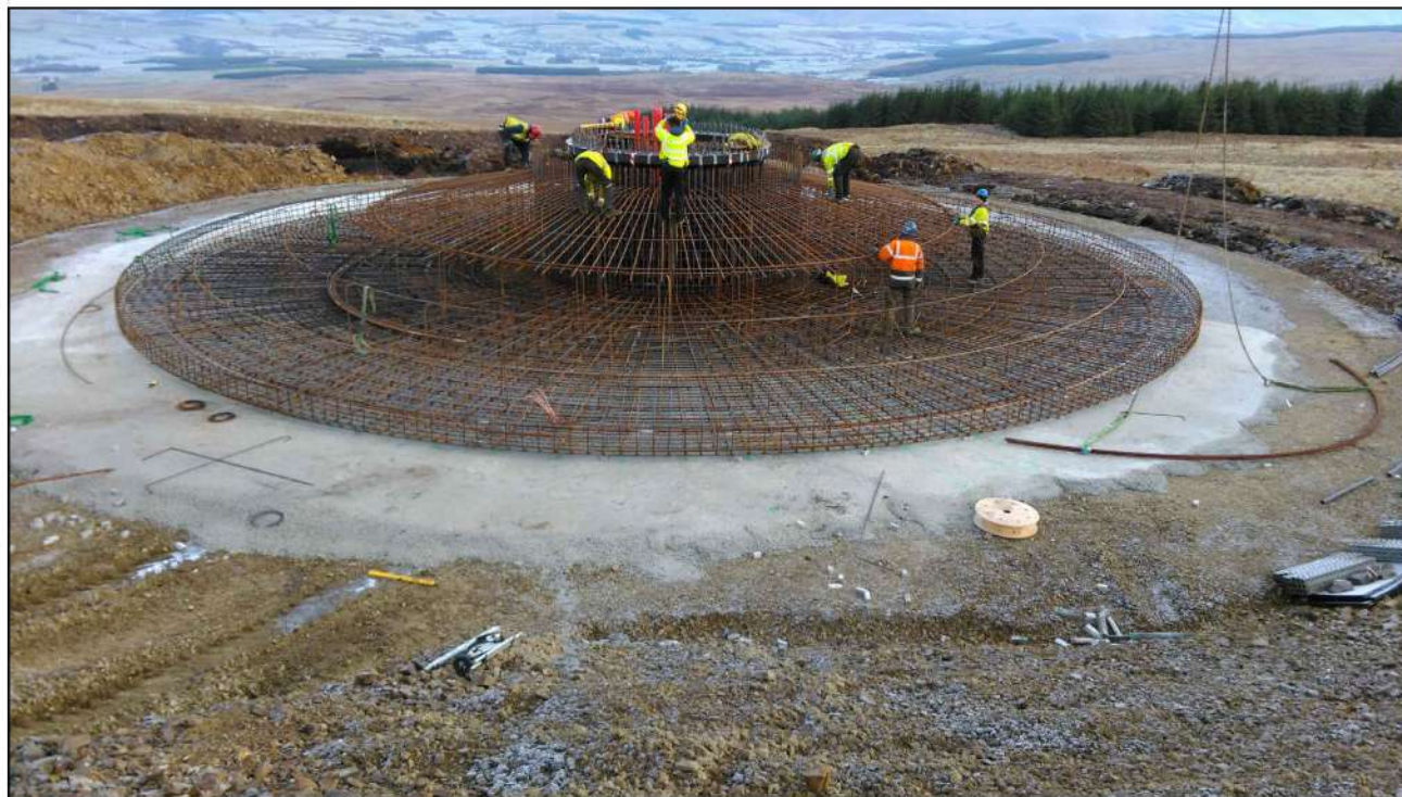
AI Plate 2.2a - Steel reinforcement which forms the turbine foundation at Sanquhar Community Wind Farm.
