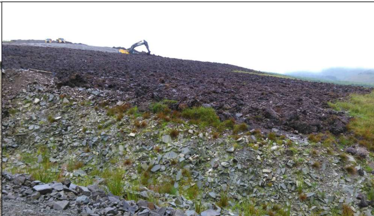
AI Plate 2. 7a - Borrow pit reinstatement at Sanquhar Community Wind Farm.
