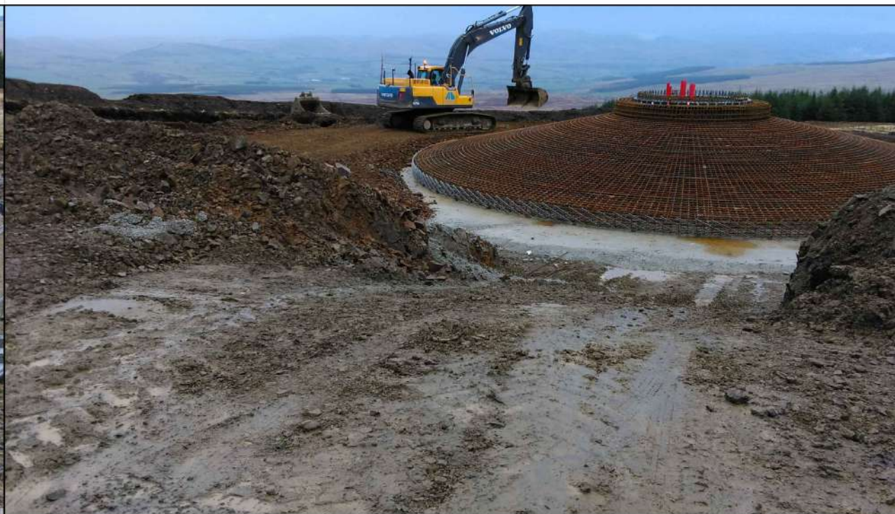
AI Plate 2.2b - Steel reinforcement which forms the turbine foundation at Sanquhar Community Wind Farm.
