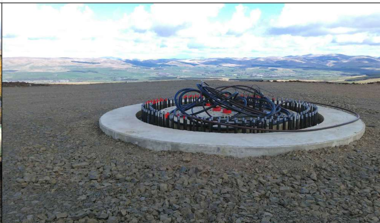
AI Plate 2.3b - Concrete finishing to a turbine foundation before backfilling at Sanquhar Community Wind Farm.
