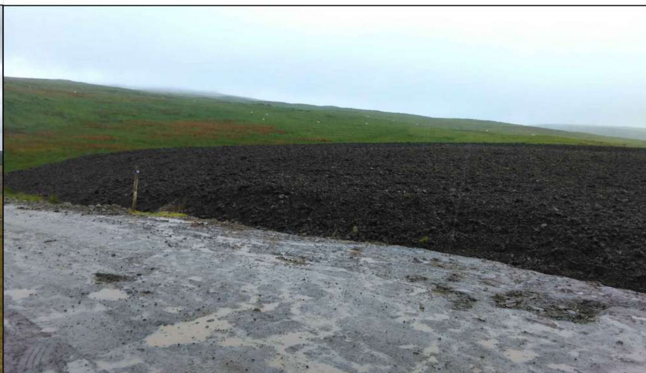
AI Plate 2. 7c - Borrow pit reinstatement at Sanquhar Community Wind Farm.
