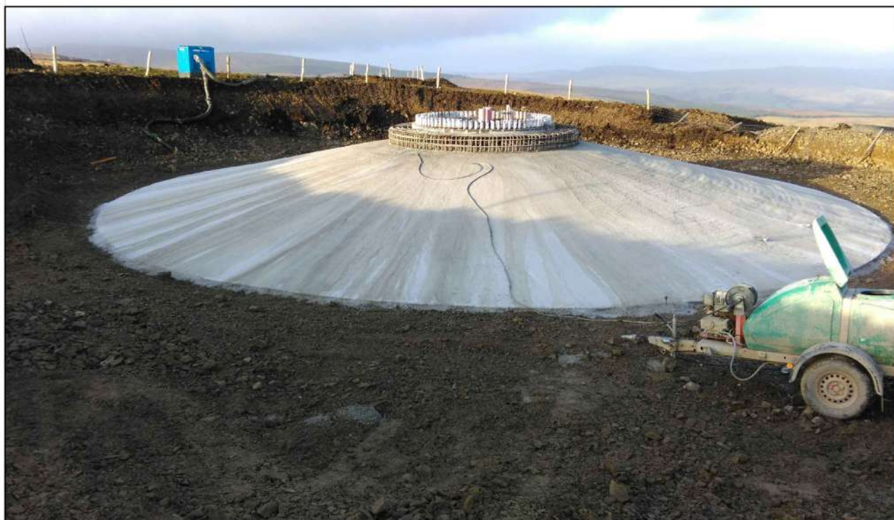
AI Plate 2.3a - Concrete finishing to a turbine foundation before backfilling at Sanquhar Community Wind Farm.
