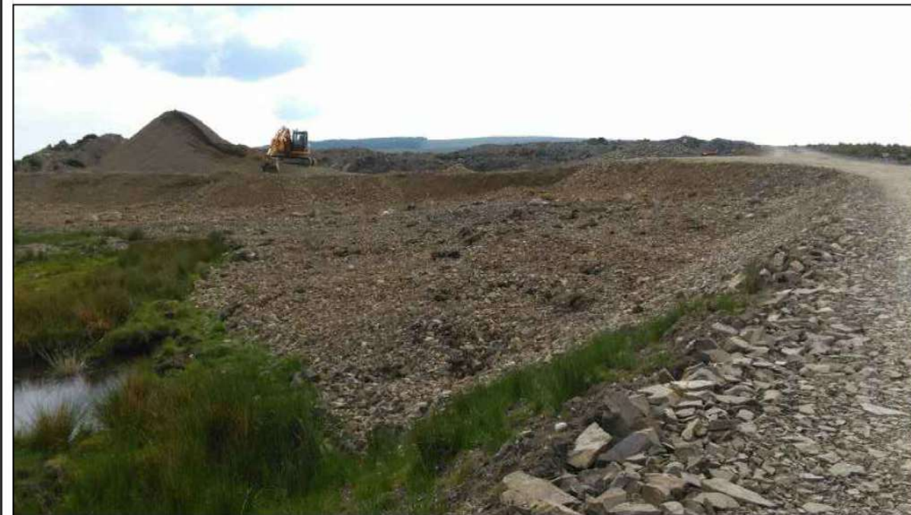
AI Plate 2. 6 - Borrow pit operation at Sanquhar Community Wind Farm.
