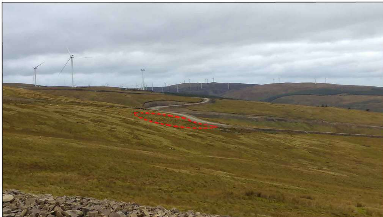
Plate 2.7b - Borrow pit reinstatement at Sanquhar Community Wind Farm
