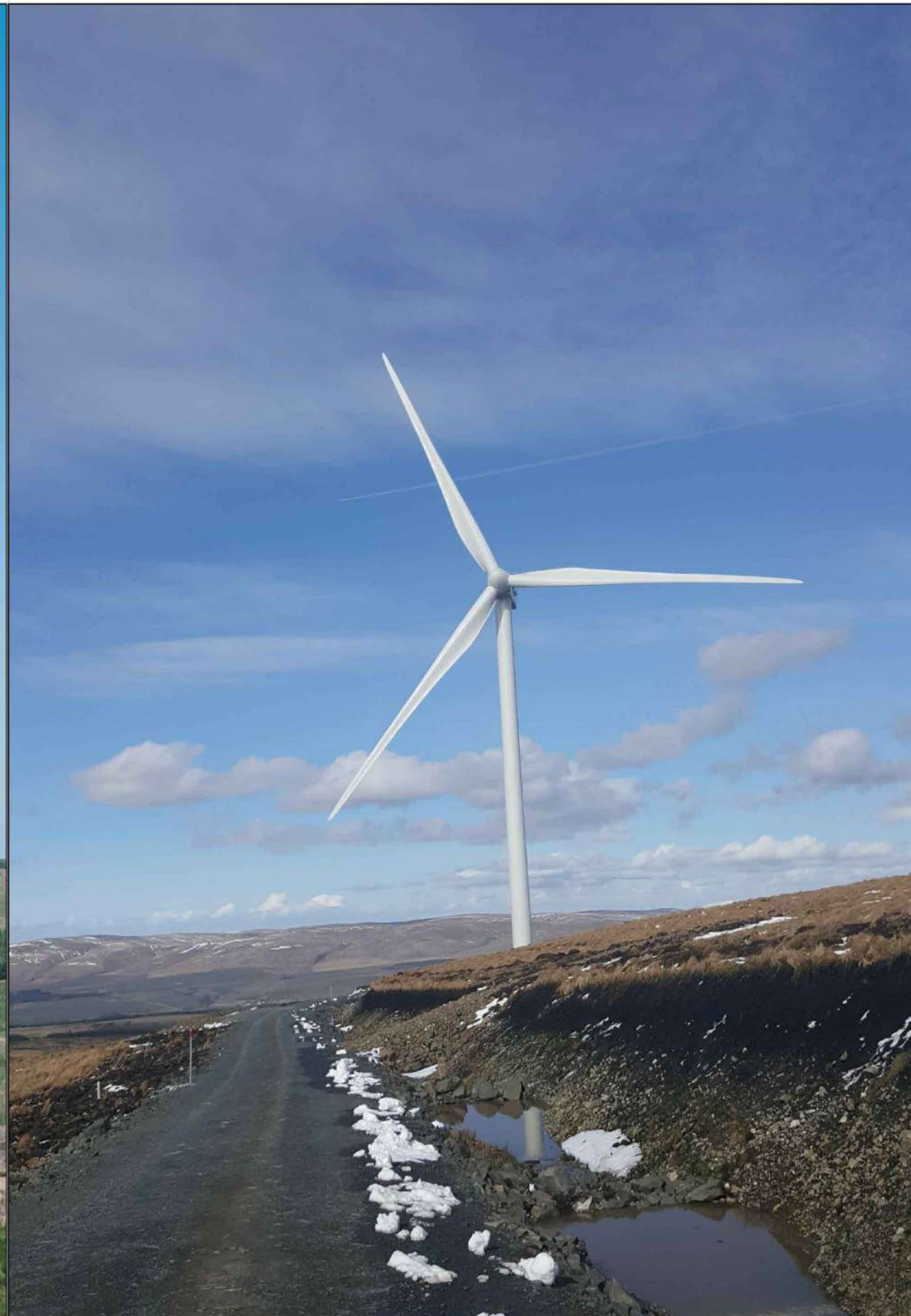
Plate 2.1b - The wind turbines installed at Sanquhar Community Wind Farm
