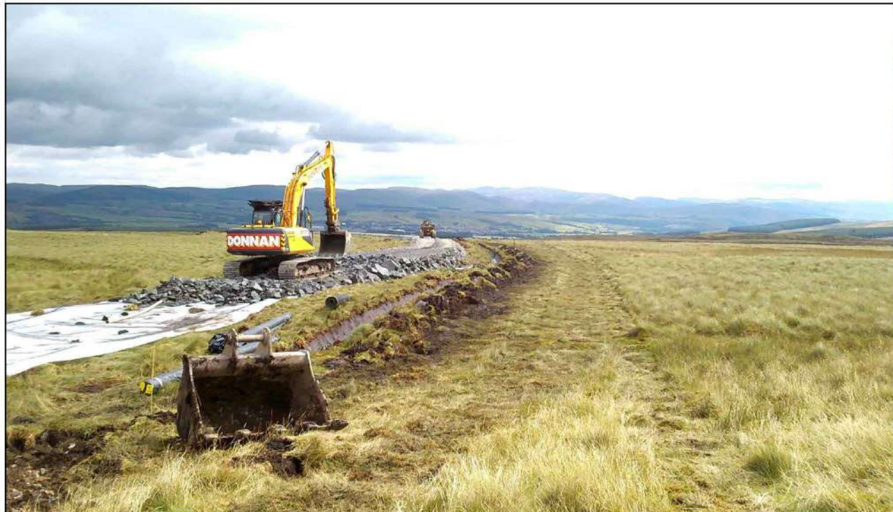
Plate 2.4a - The construction of a floating road at Sanquhar Community Wind Farm
