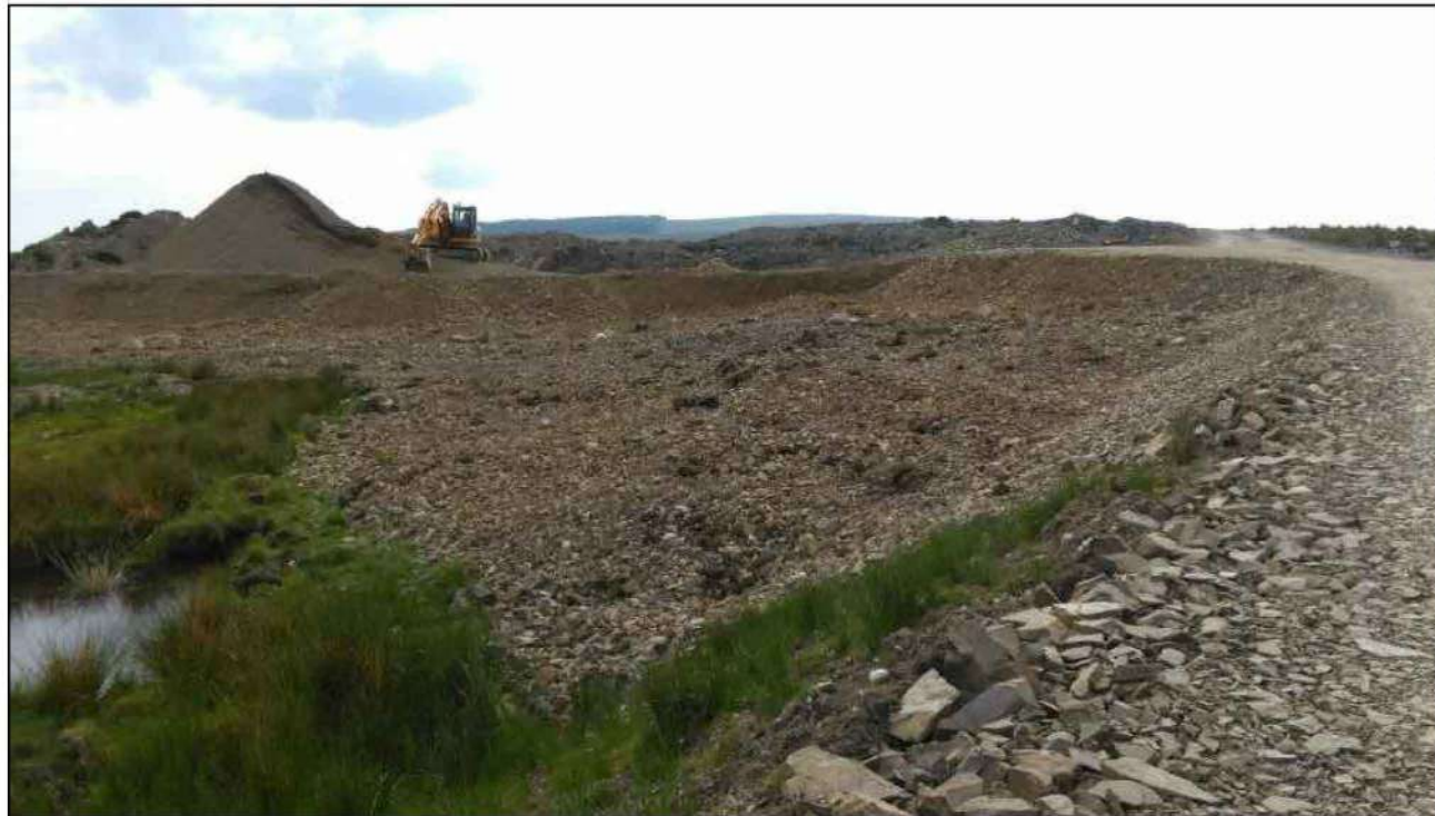
Plate 2.6 - Borrow pit operation at Sanquhar Community Wind Farm
