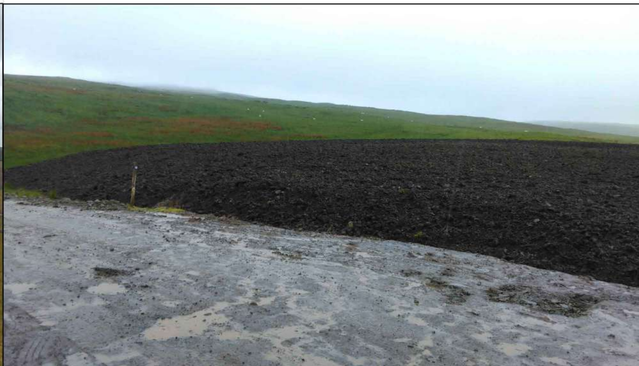
Plate 2.7c - Borrow pit reinstatement at Sanquhar Community Wind Farm
