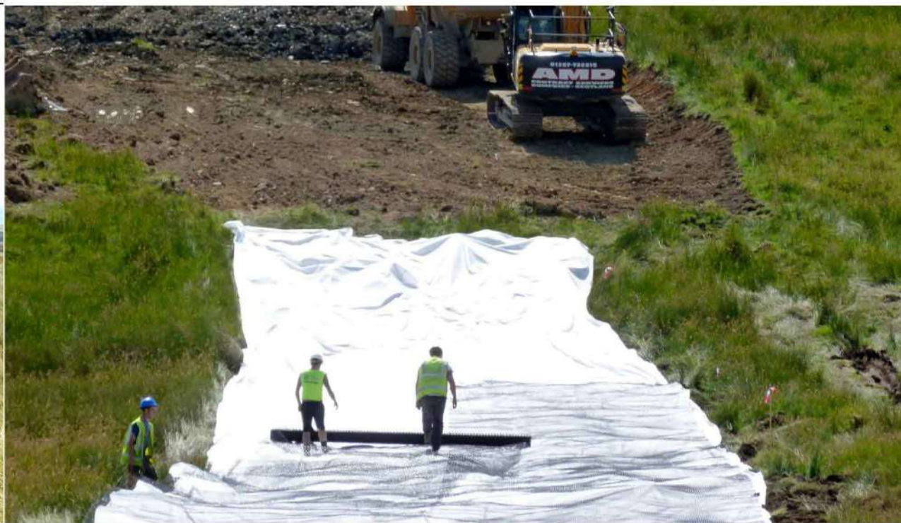
Plate 2.4b - Floating track into cut track transition at Sanquhar Community Wind Farm
