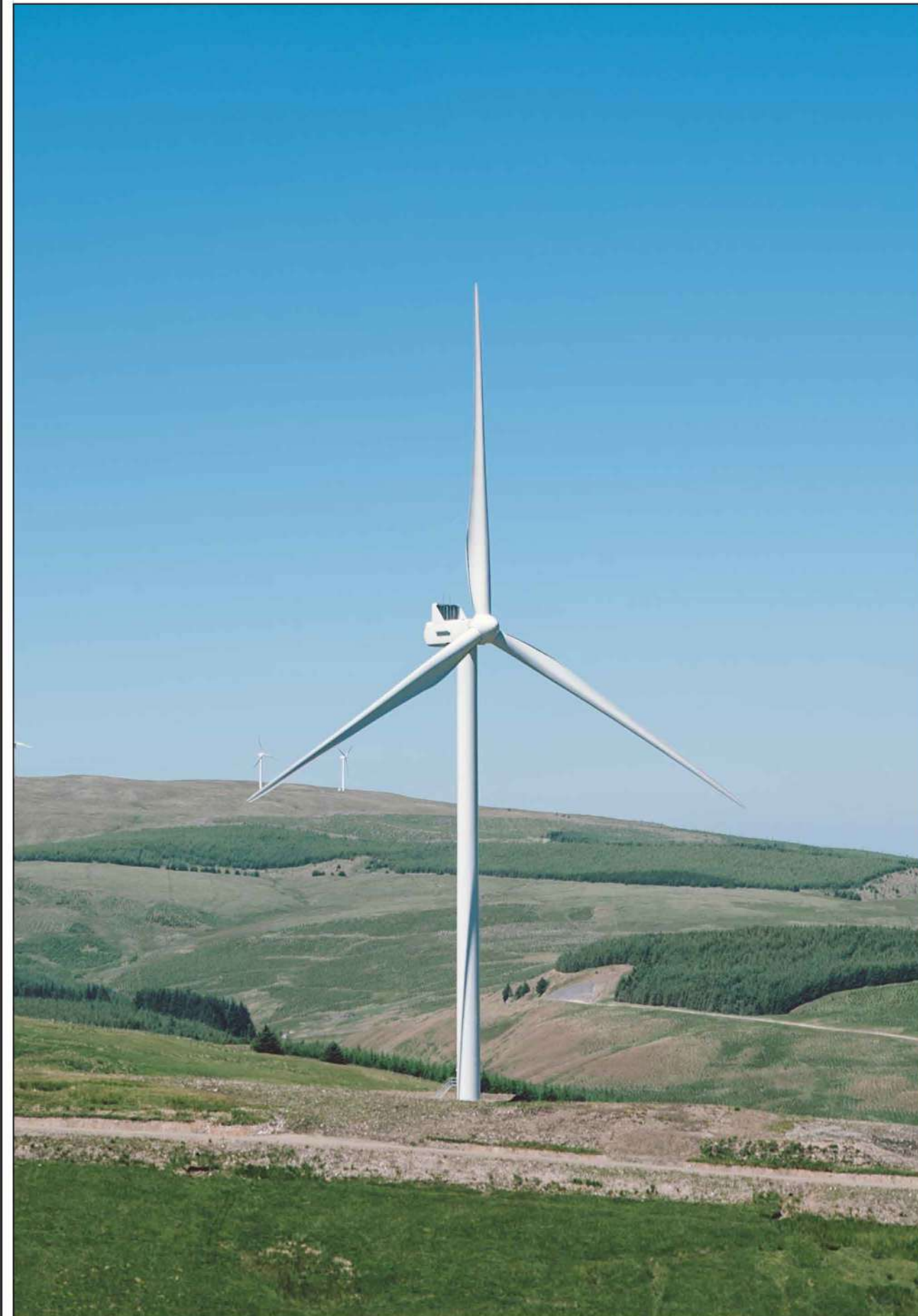
Plate 2.1a - The wind turbines installed at Sanquhar Community Wind Farm
