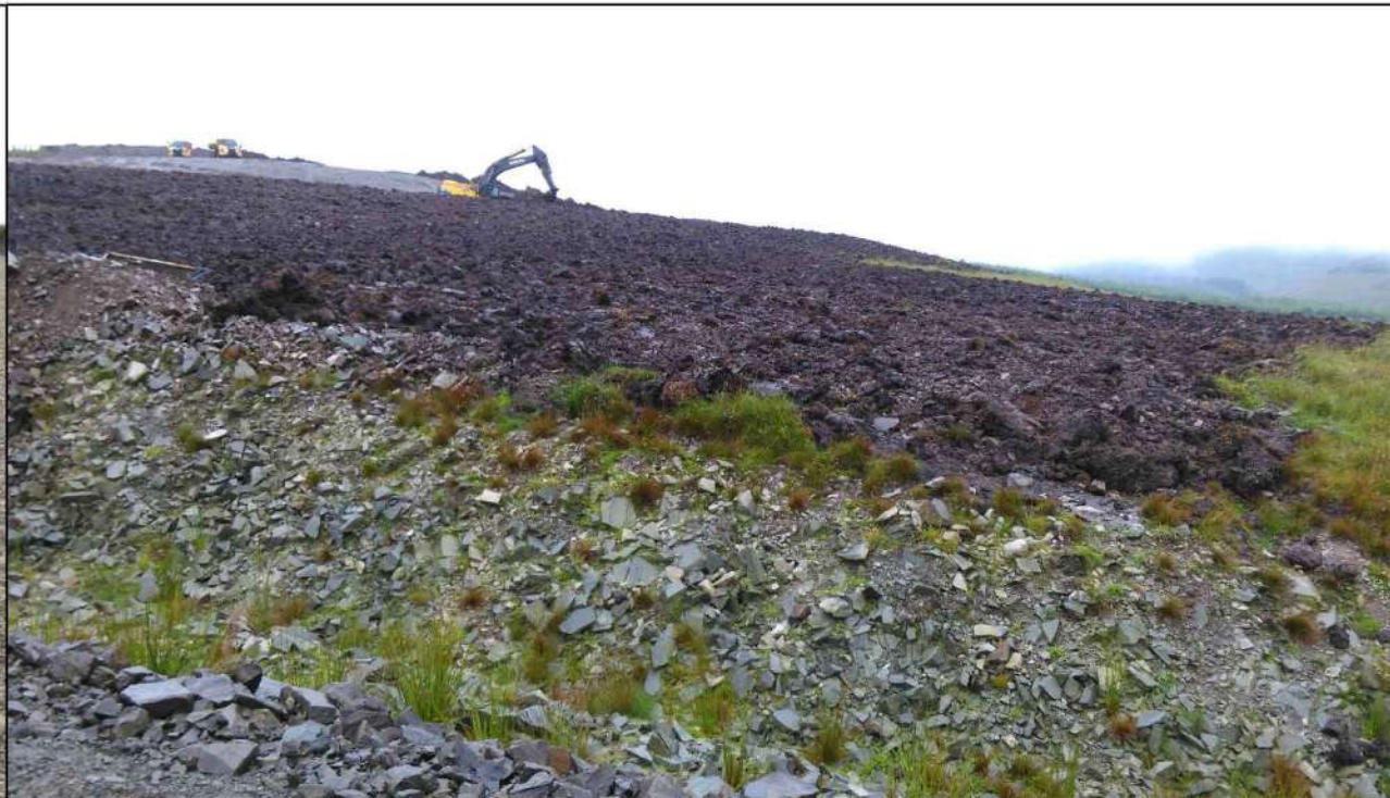
Plate 2.7a - Borrow pit reinstatement at Sanquhar Community Wind Farm
